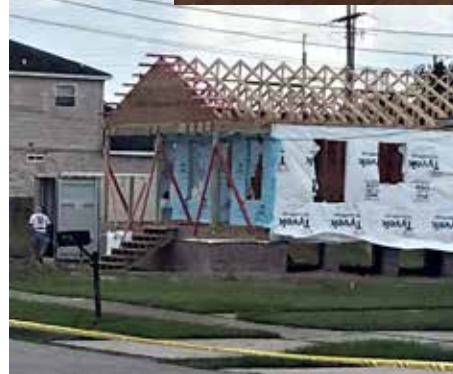
3rd House: Built interior walls!
