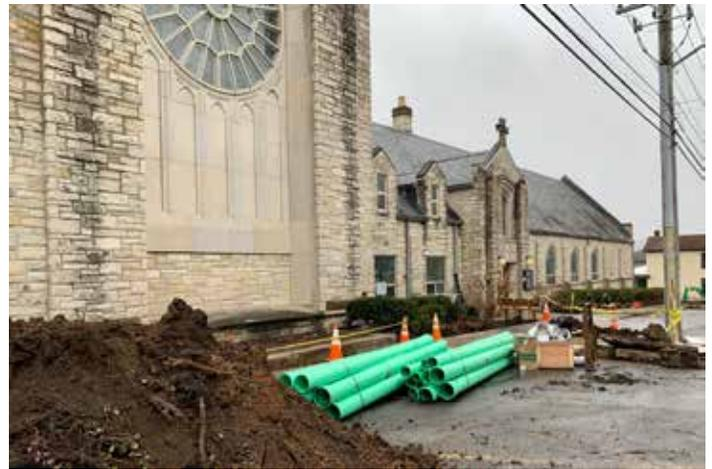
What was all that digging about? Some long needed drainage improvements were recently completed on the Cedar Street side of the building. Until now, the downspouts from our roof have drained across the sidewalks and into what is now our handicapped accessible parking. A drainage system was installed along the full width of the system to drain the downspouts into the city's drainage system.
